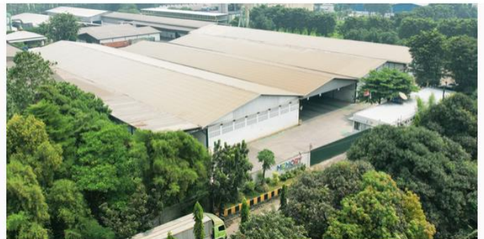
Panel Production Plant
