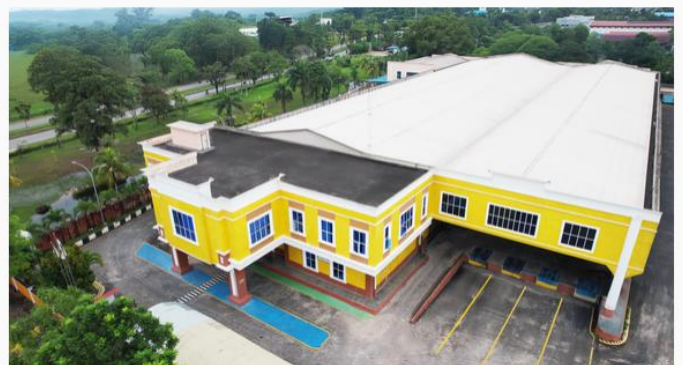
Panel Production Plant
